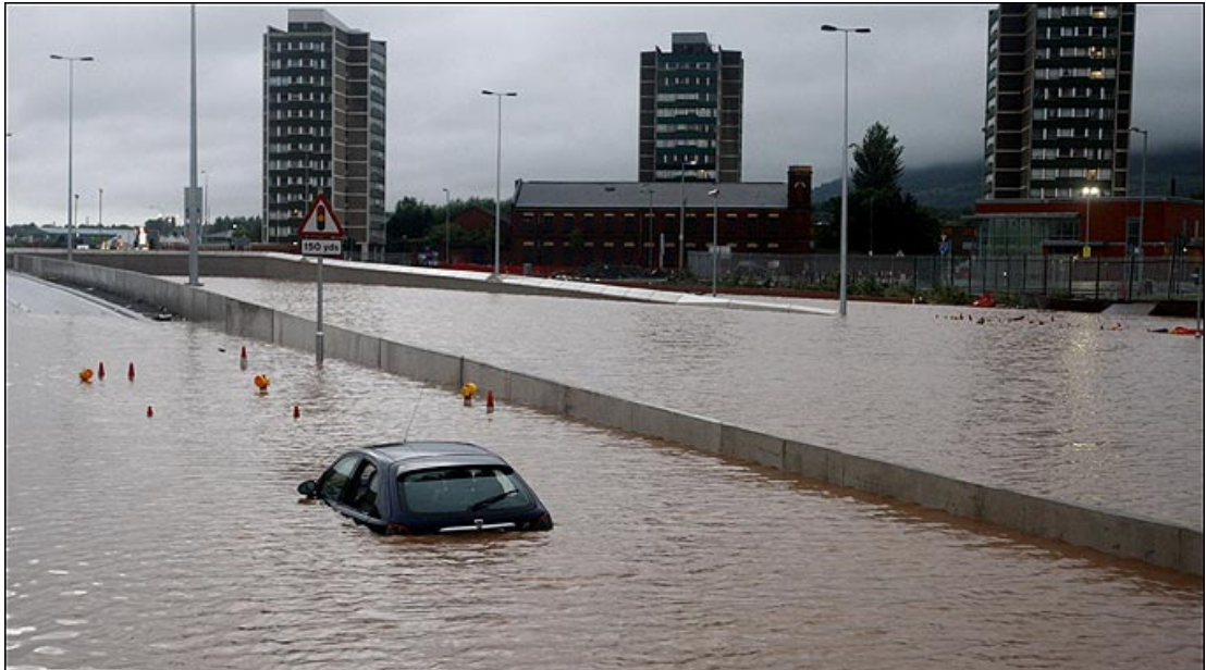
Figure 3 Flooding at Broadway Underpass
